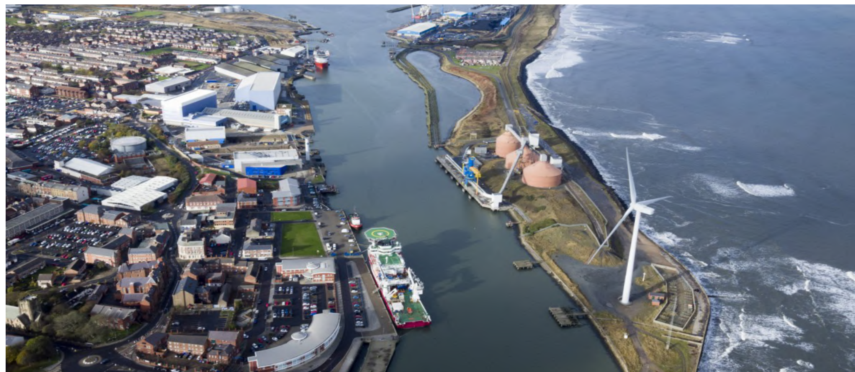
AERIAL IMAGE OF PORT OF
